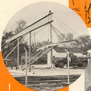
Steel building sections are raised simply, easily with the power winch.
