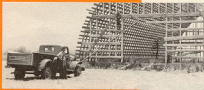
In construction work, the Power-Wagon is used for many moving, hoisting and pulling operations. It brings its own "power plant" right to the job.
